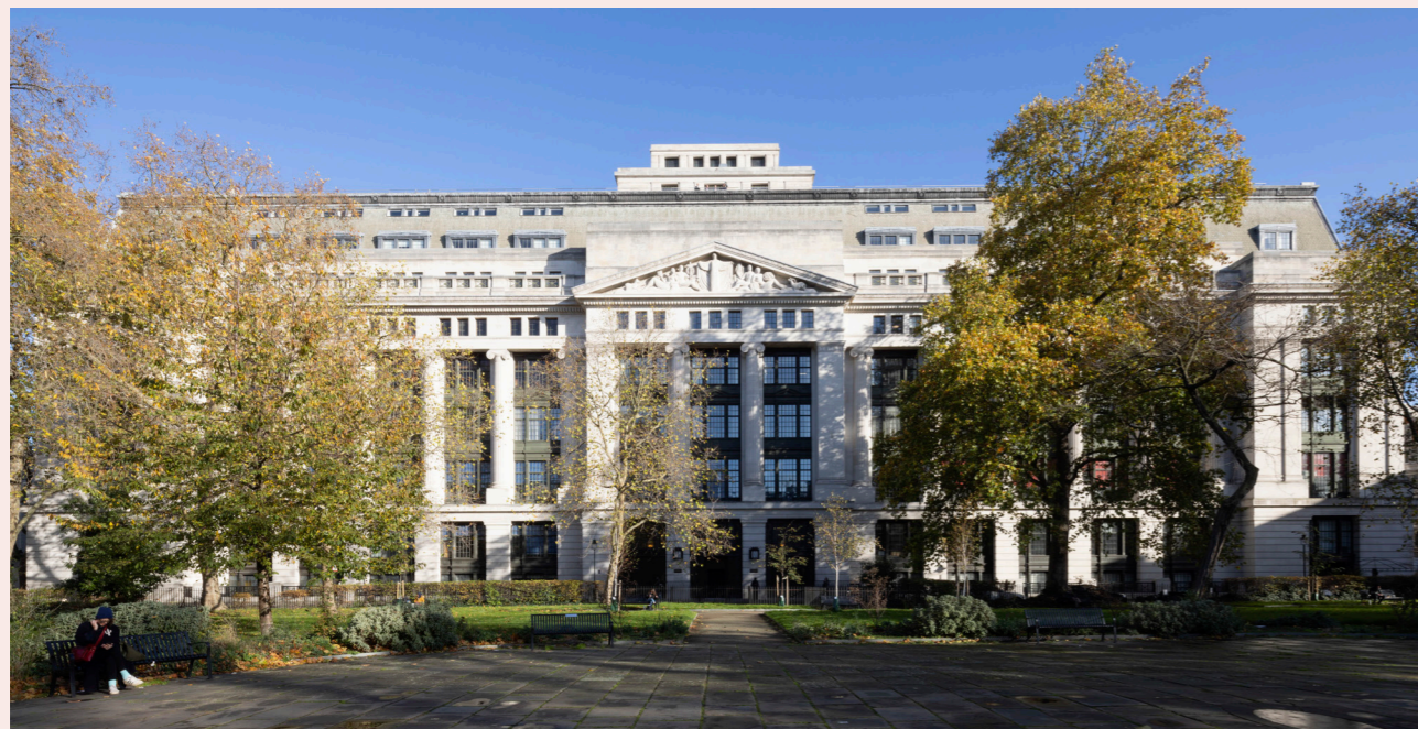
Victoria House, Oxford Properties and Pioneer Group
