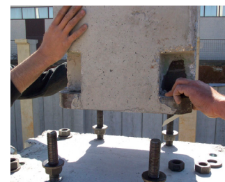
Prefabricated concrete pillars are mounted using Peikko pillar shoes.
