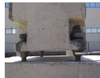
Attachment and adjustment of the elements can easily be done by means of a wrench.
