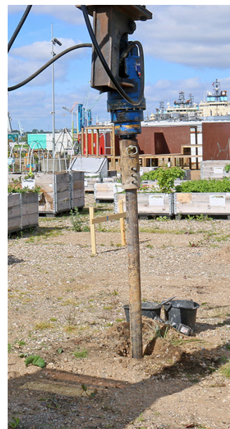
Screw piles are installed with construction machinery.
