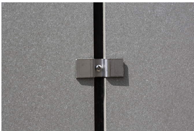
The wing fasteners are attached with one screw.
